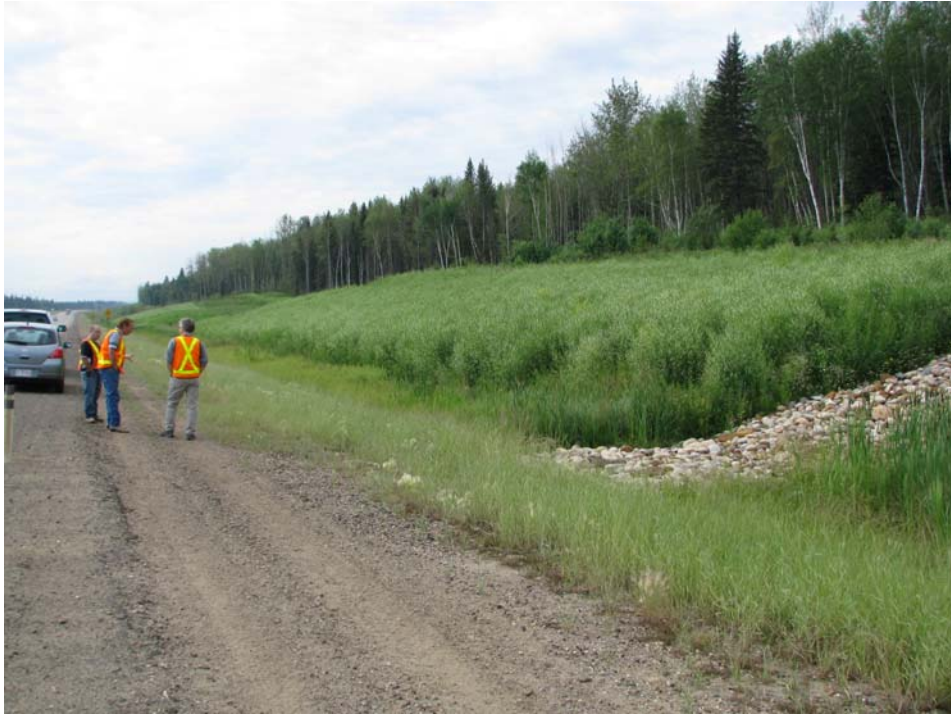
Photo 1 - North Slump, looking south (July 8, 2008).
