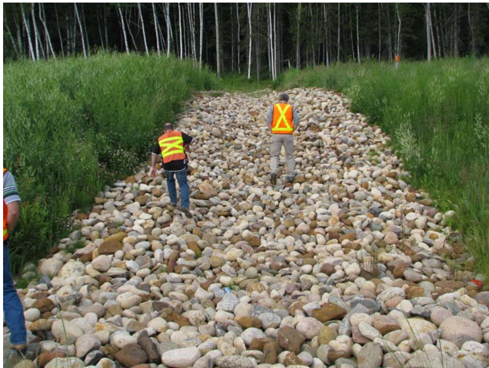
Photo 2 - North swale (July 8, 2008).
