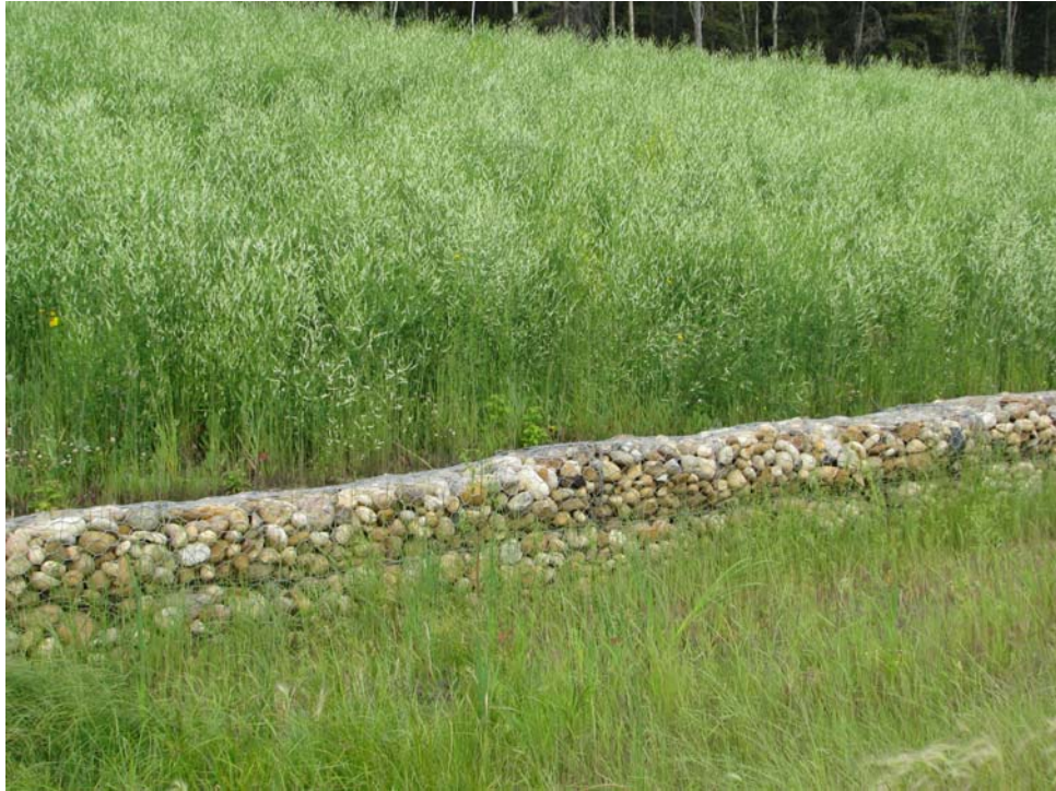
Photo 7 - Looking west at the South Slump repair (July 8, 2008).
