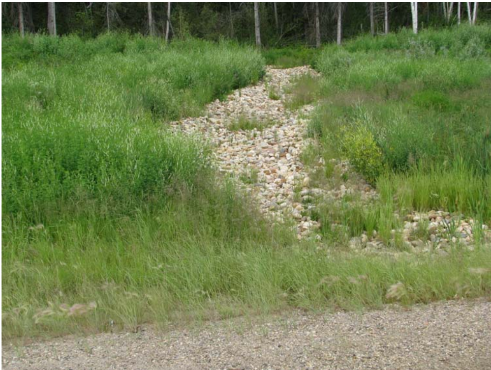
Photo 8 - South swale (July 8, 2008).
