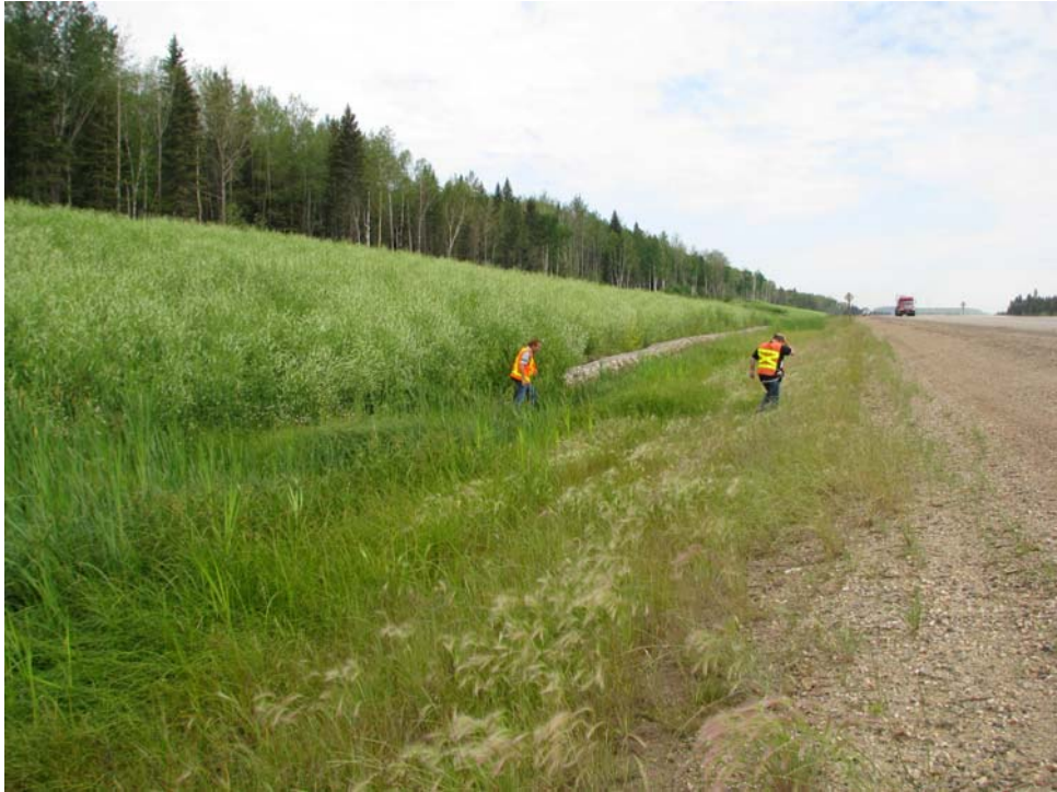
Photo 5 - Looking northwest at the South Slump repair (July 8, 2008).
