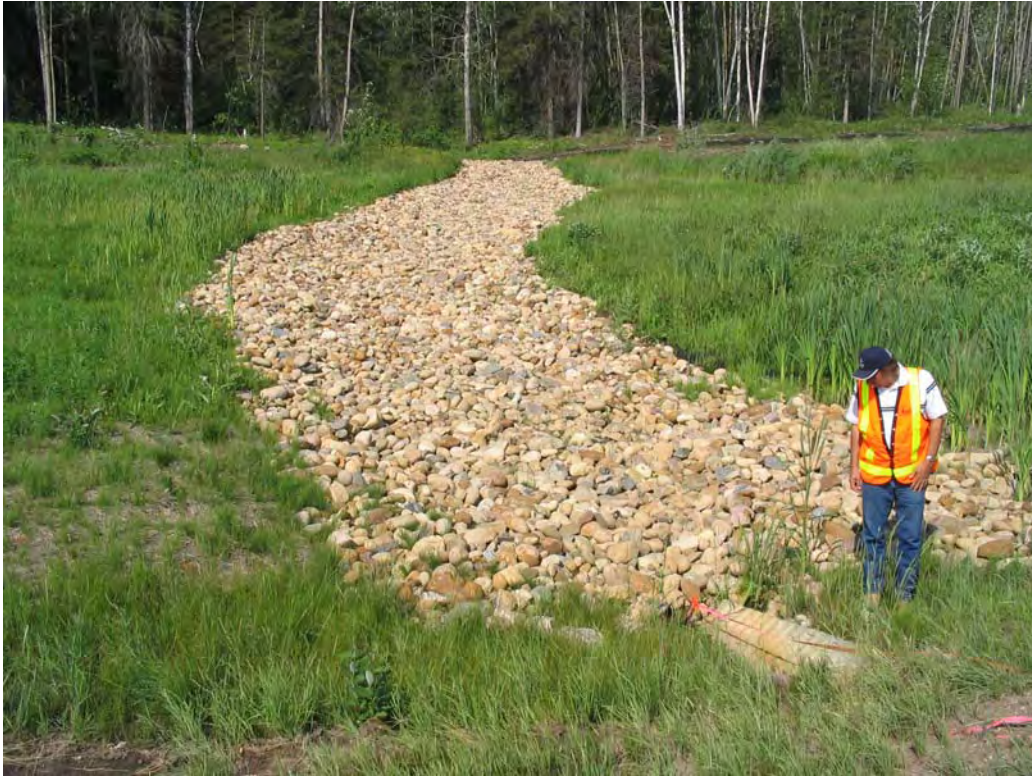
Photo 5 - Armoured Swale Between the Repaired Slump Areas.
