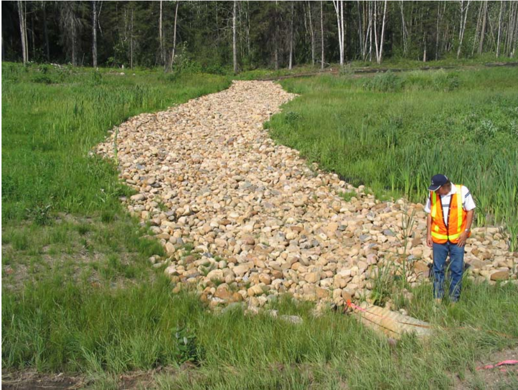
Photo 5 - Armoured Swale Between the Repaired Slump Areas.
