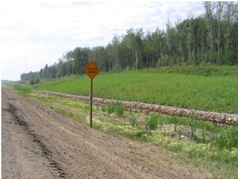
Photo 2 - Repaired South Slump Area.
