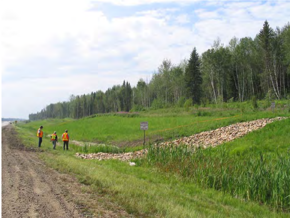
Photo 1 - Repaired North Slump Area and swale.
