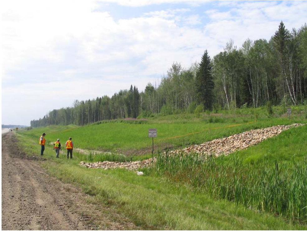
Photo 1 - Repaired North Slump Area and swale.
