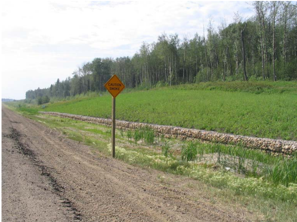
Photo 2 - Repaired South Slump Area.
