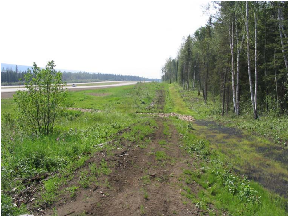
Photo 4 - Catchwater Ditch and Shallow Berm at Top of Cleared Slope.
