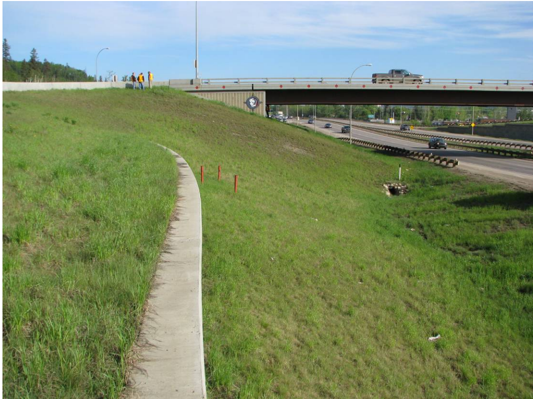
Photo #1 General view of the west side of the bridge (looking northwest)
