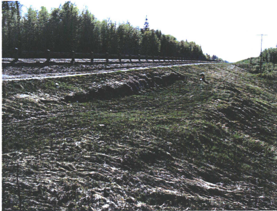
Photo 1 - Looking west at the distress area, May 24, 2007.
