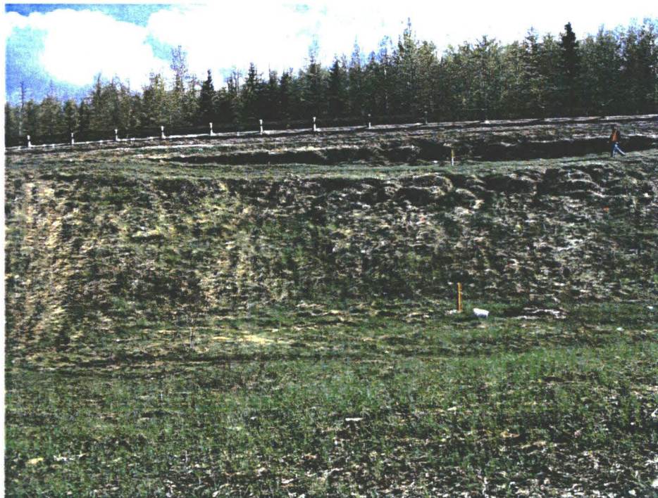
Photo 4 - Looking south at the side slope area (SI's), May 24, 2007.
