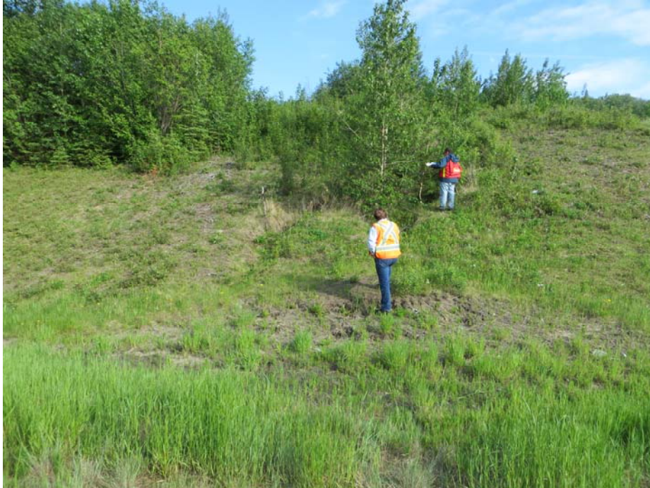
Photo# 1 General view of highway backslope slump; note that vegetation has grown within the slump mass (looking south)
