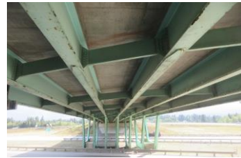
Rolled Beam with Cover Plates
