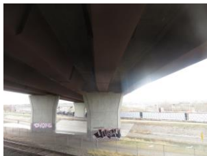
Steel Tub Girders
