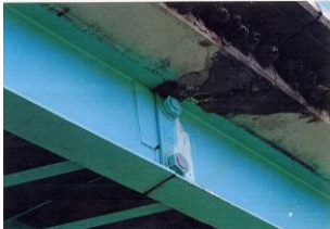
Girder with Pin & Hanger
