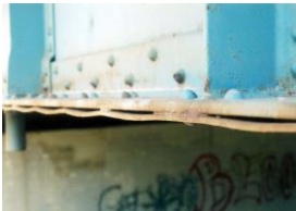
Rippling of Plate
