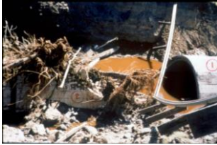
Centre section of the culvert
