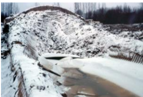
Inlet with culvert still connected to headwall
