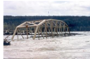
One span tipped in middle channel and other one around near shore.
