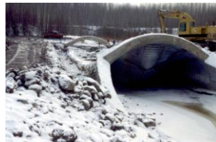
Overview of culvert inlet
