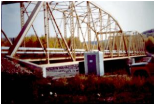
Bridge built in 1982, 122m bridge
