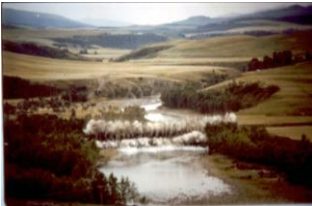
Removing the bridge in August 1980
