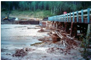
Forestry bridge built in 1960, 380 ft. long bridge
