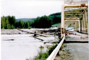
Bridge floating and starting to shift
