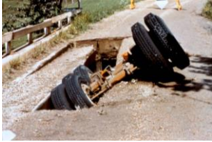
Pup tandem axle in hole left by dropped girder
