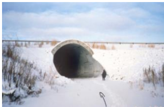
U/S inlet of new culvert
