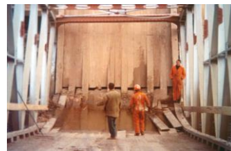
Abutment end of the bridge showing timber decking etc.
