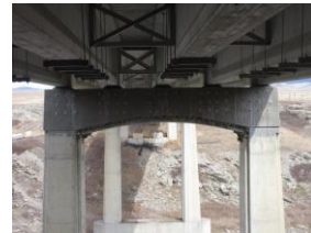
BF 1153 – Neoprene Pads & Widened/Strengthened Pier Caps
