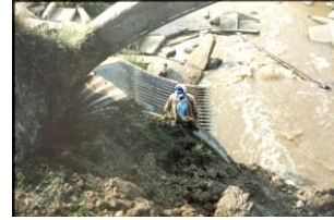
Outlet of culvert
