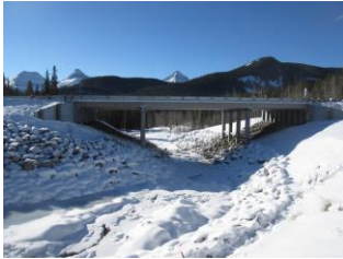
BF 77496 – Replaced in 2015 with new 8-14-8 M SLW girder bridge
