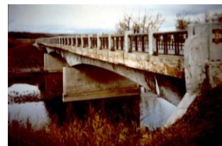
Bridge condition in 1979 (28 years old)
