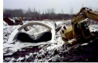
Outlet showing intact end treatment
