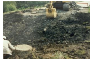
Water and sewer line in embankment
