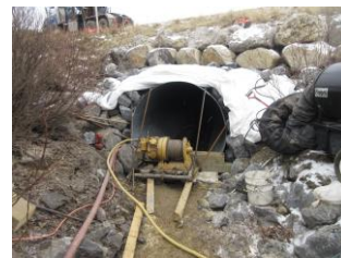
Winch at Outlet to pull new CSP liner into pipe
