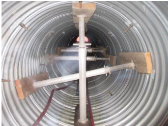
Internal Bracing Installed Prior to Grouting
