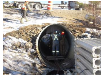
Installing Steel Headwalls at Ends of Pipe to contain grout
