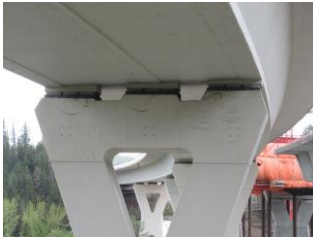
Multi Pot Bearings - Expansion
