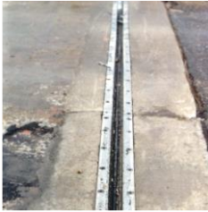
“Honel” Gland Joint with Bolted Compression Connection
