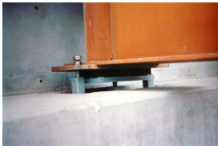
Elastomeric Bearing Showing Pintel, Anchor, Bolts, Sole and Masonry Plates (before grouting)
