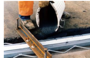
Placing Wabocrete Two Component Elastomeric Material
