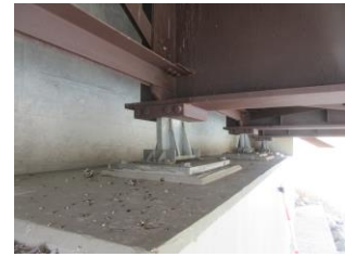
Rocker Bearing Under Steel Girder
