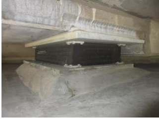
Reinforced Neoprene Bearing without Teflon & Stainless Steel
