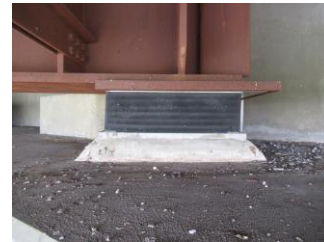
Reinforced Neoprene Expansion Bearing with Teflon & Stainless Steel
