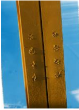
All verticals have plug welds at original sway brace bolt location.
