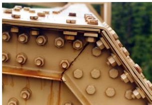
All USN, bevel faying fit is torched. Reduced edge distance
