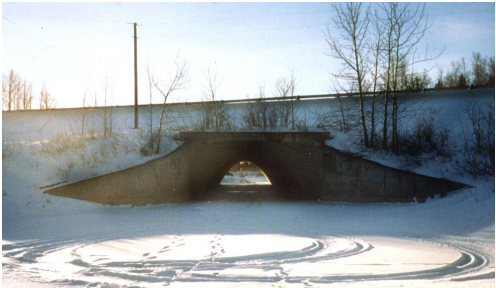
Concrete arch culvert with curved wingwalls in Feb. (Weed Creek)
