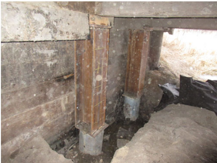
Timber Piles Repaired with Steel Splice
