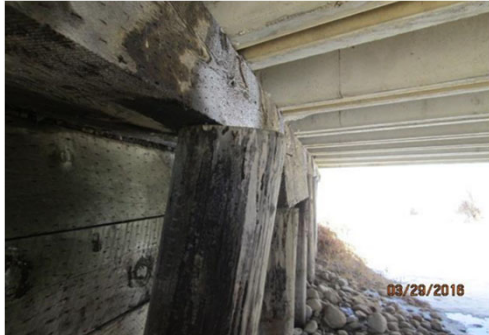
Timber Pile Not Sharing Load – Rated 3
