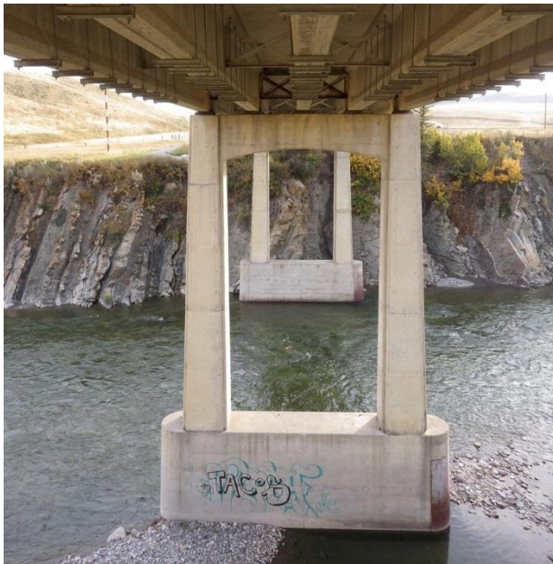
Figure 3: Concrete pier with shafts and arched cap.
