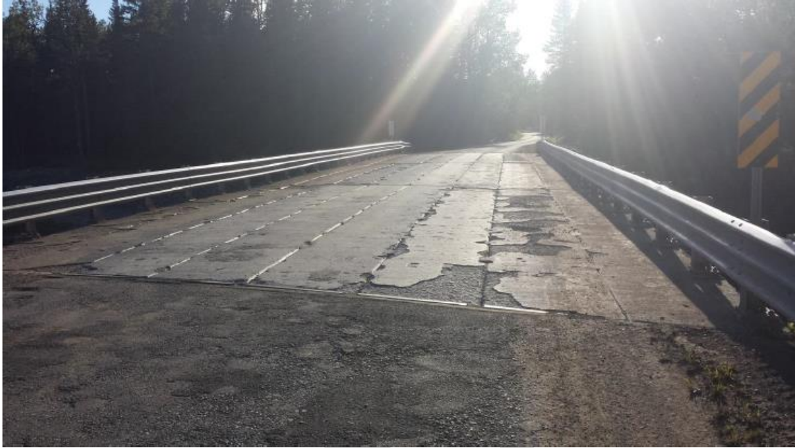
Example 3: Section loss along top corners and top surfaces of interior girders. Interior girders rated 3.
