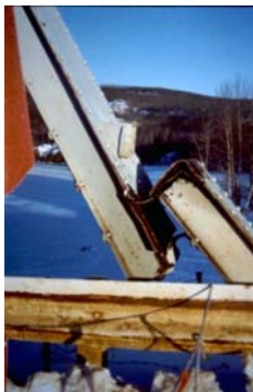
Severed batter post U7 - L8
