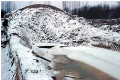
Inlet with culvert still connected to headwall
