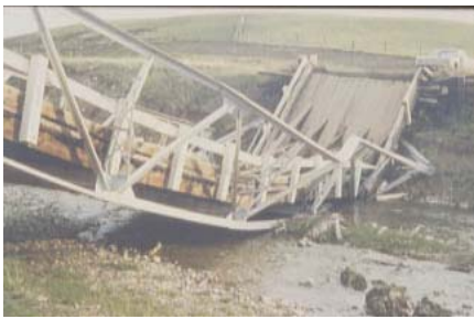
Overload Damage
