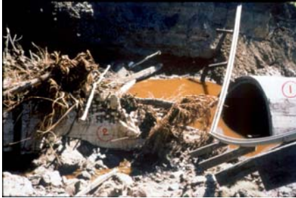
Centre section of culvert
