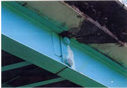
Girder with Pin & Hanger
