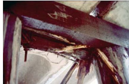
Failed pier cap with girder dropped to pile top level
