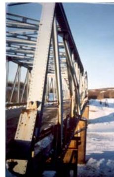
Broken hanger U7 - L7 and first diagonal U7 - L6
