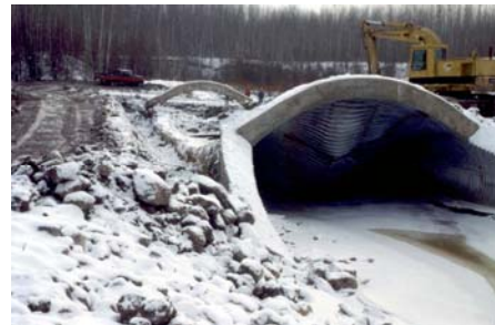
Overview of culvert inlet
