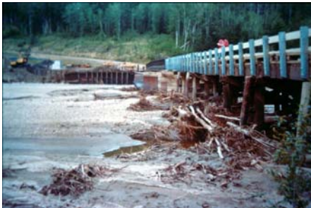
Forestry bridge built in 1960, 380 ft. long bridge
