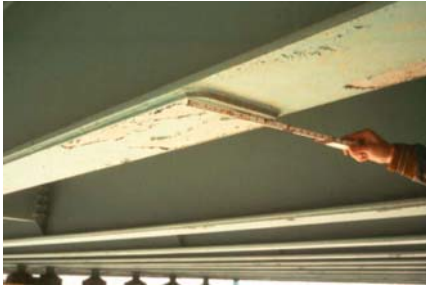
Rolled Beam with Cover Plates
