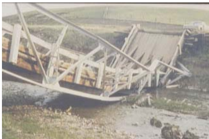
Overload Damage
