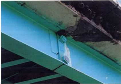
Girder with Pin & Hanger
