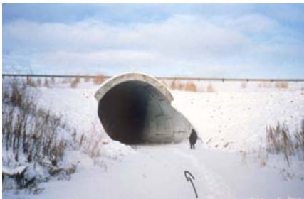
u/s inlet of new culvert
