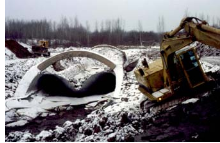
Outlet showing intact end treatment
