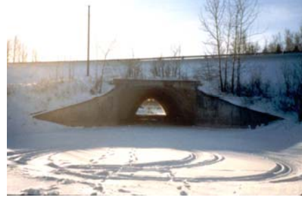
Concrete arch culvert in 1989
